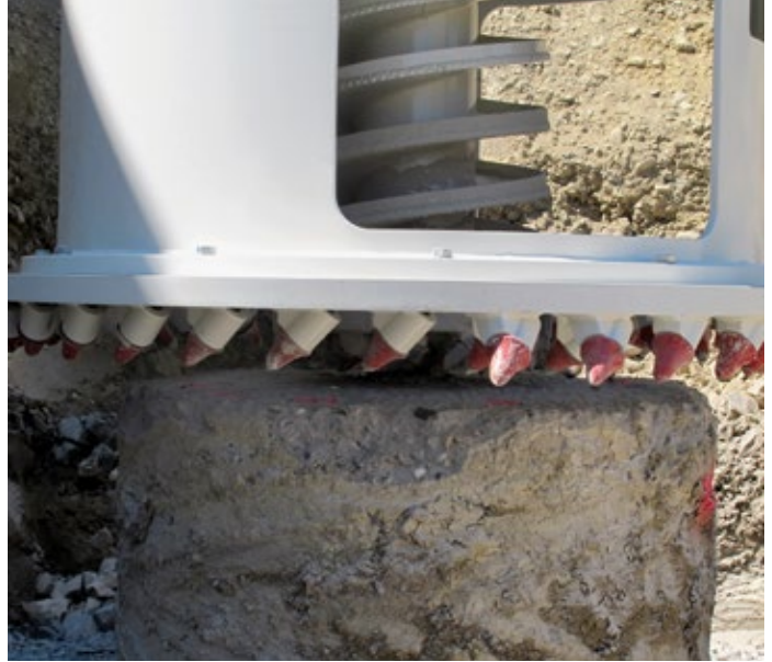
In a first phase, the milling disc is used to remove the pile head down to the reinforcement bars (left picture). In a second process step, the inner cutter breaks the core tension, the outer cutter simultaneously breaks the surface tension of the concrete (right picture).
