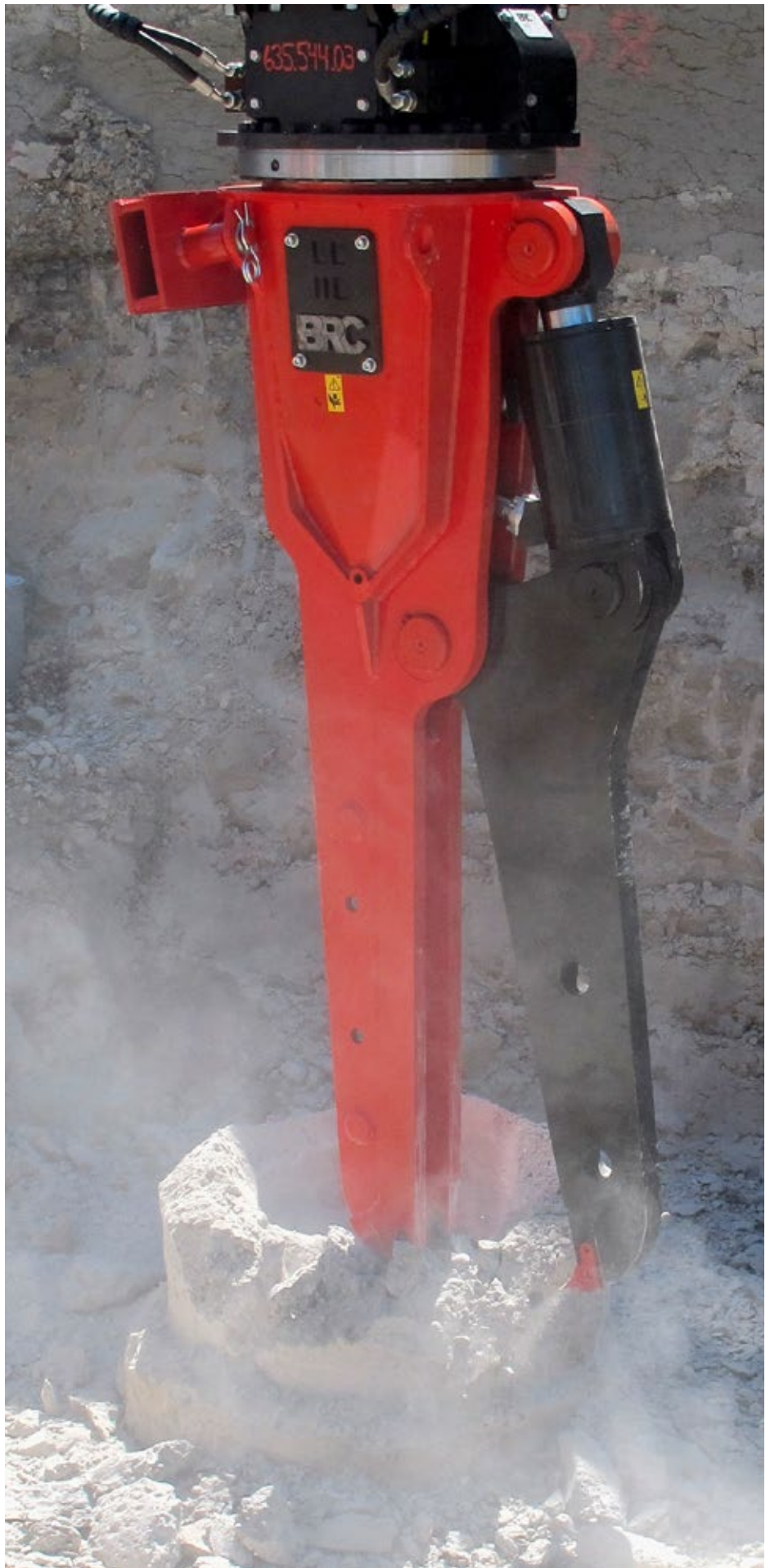
The Brextor system's drill head and biters are 1.8 metres long. This means that reinforcements can be exposed up to an appropriate height so that the length of the connecting reinforcements meets the standards of earthquake safety.
