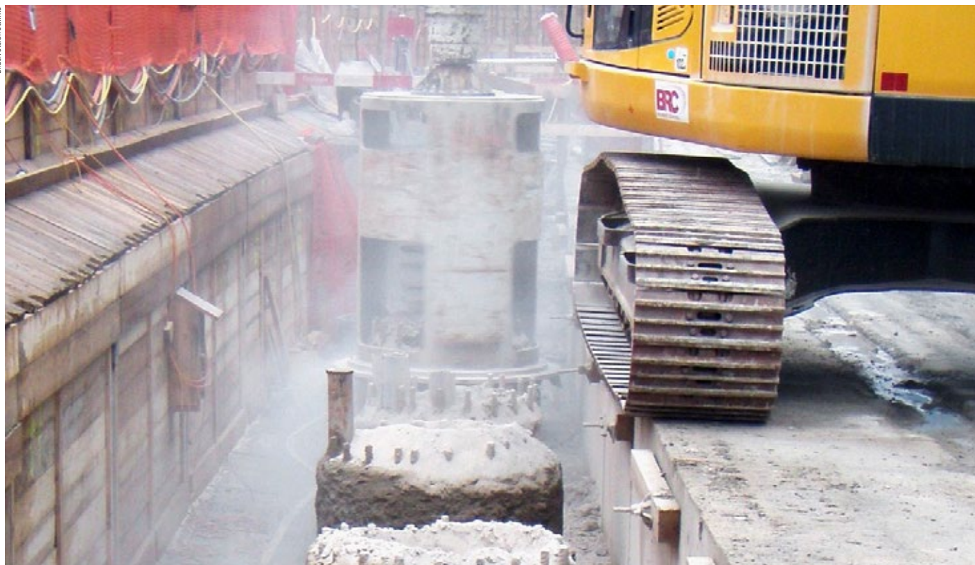
Milling inside and outside at the same time is part of the well thought-out principle of the Brextor.
